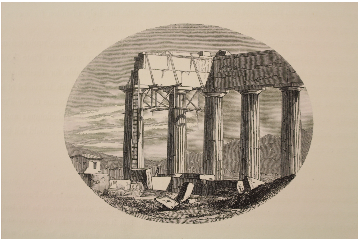
Abb. 7 Vermessung des Parthenon, Vignette aus Francis Cranmer Penrose, An Investigation of the Principles of Athenian Architecture , London 1851
